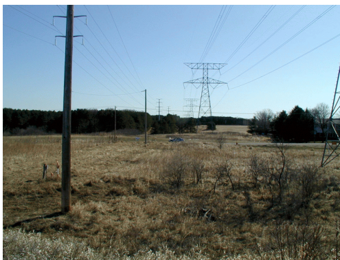
Photo 15 – looking east along the powerline easement from the Bruce Vento trail/NSP substation area.
