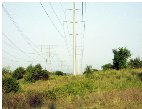
Photo 10 – looking west from McKnight into the public open space and along the powerline easement.
