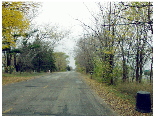
Photo 7 – looking west along County Road “D”, which illustrates the limited width of the existing road (23') and adjacent R.O.W.
