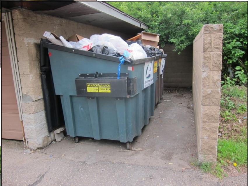
Undersized enclosure – trash only (recycling less convenient)
