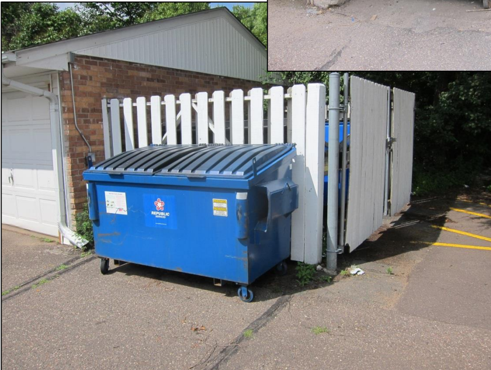
Undersized enclosure – recycling next to trash enclosure (recycling more convenient)
